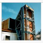
Donaldson designs and produces customized inlet cooling systems, such as evaporative coolers and chiller coils. These systems provide additional power output from gas turbines operating in warm climates. In addition, our patented silencers provide advanced acoustical attenuation of the noise generated by the gas turbines.
